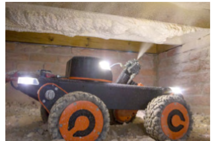
Q-Bot installs underfloor insulation
